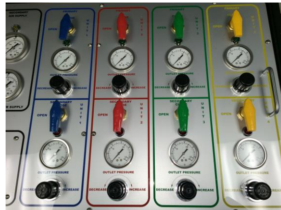
Primary and Secondary air controls
